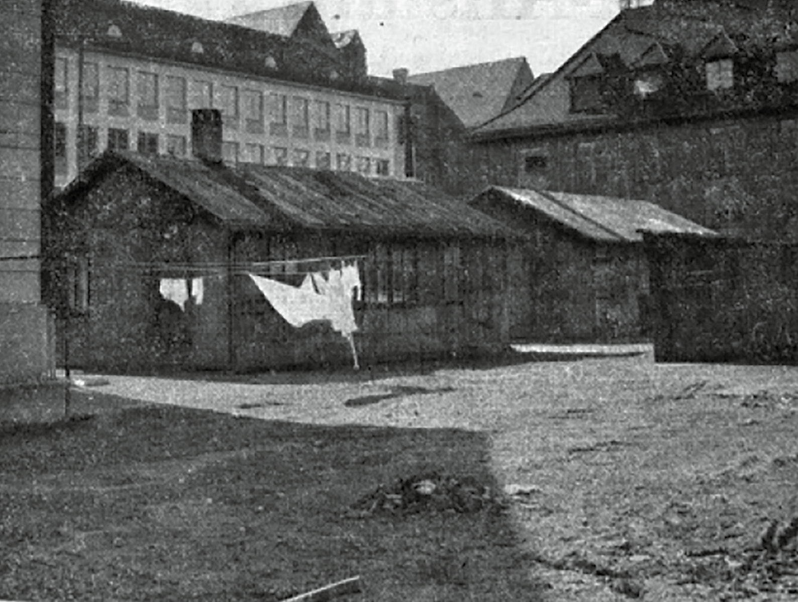
Barracks of the "Office for Emergency Housing", Neue Zürcher Zeitung, No. 502, 21.3.1956
